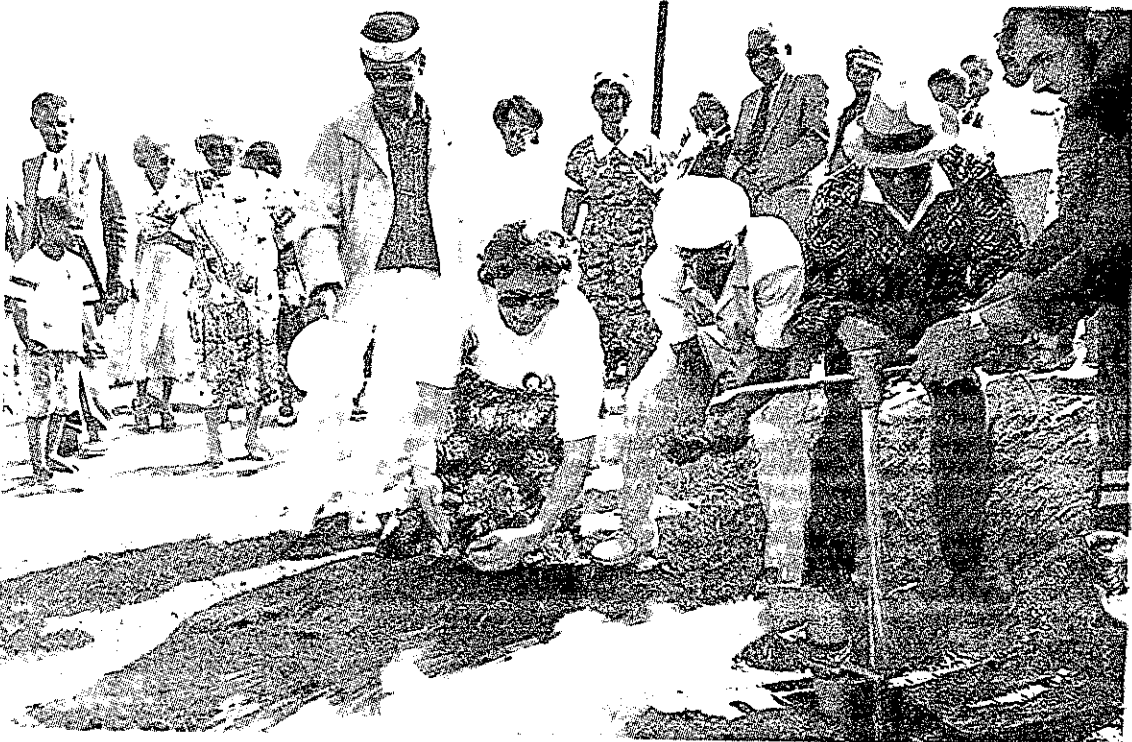
LET IT FLOW! Delighted Buisplaas residents taste the first gush of clean water flowing through the new pipeline to their historic community.
