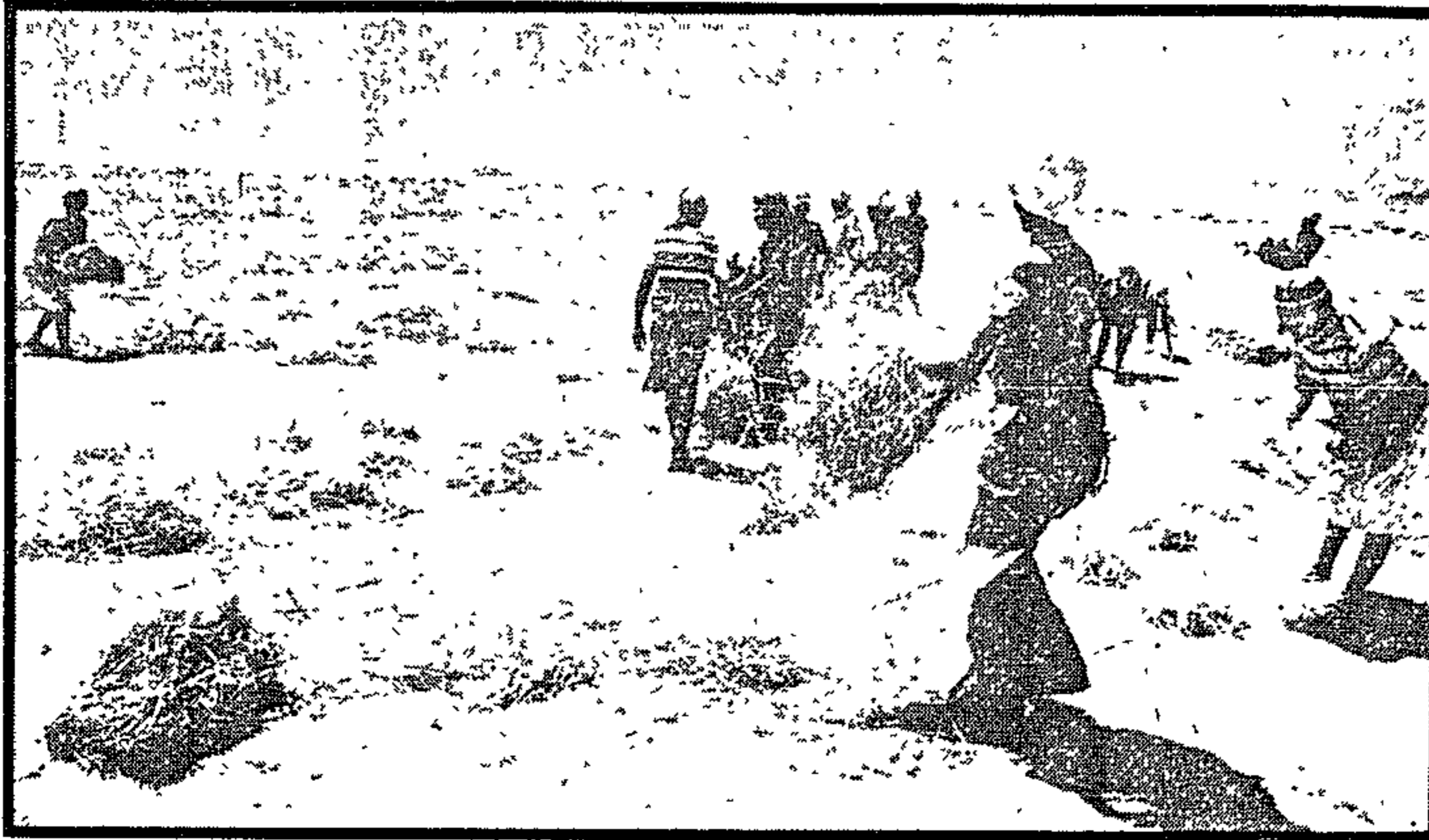
The vast tract of land being cleared for the site-and-service stands. After the earthmovers have levelled the dunes, these women come to spread straw by the bale. A tractor follows, ploughing it in to stabilise the drifting sand.
