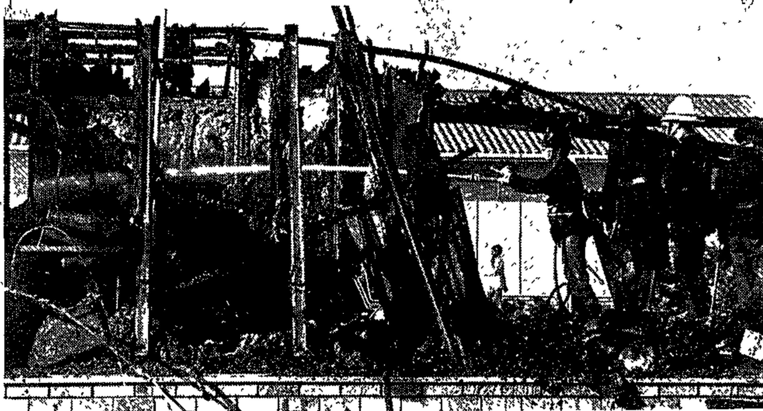
Firemen spray the last jets of water on the charred ruins of part of the Heideveld Primary School yesterday. The fire is believed to be the work of arsonists.
