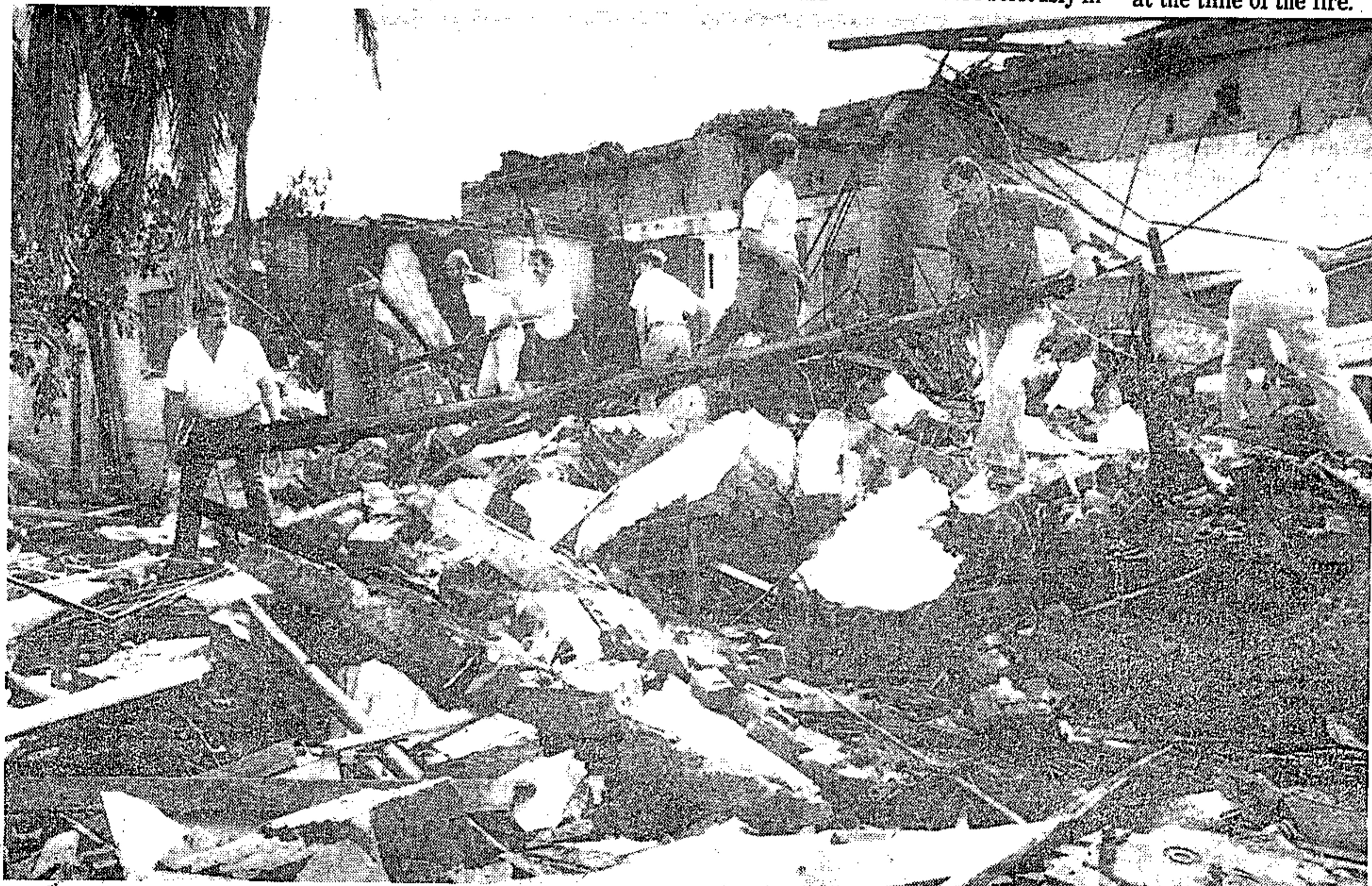
Police today combed the rubble and soot-blackened remains of the luxury Park Drive, Port Elizabeth, home of the Watson family, searching for clues to the fire which gutted the house on Saturday night. The house was insured. An arson docket has been opened.
