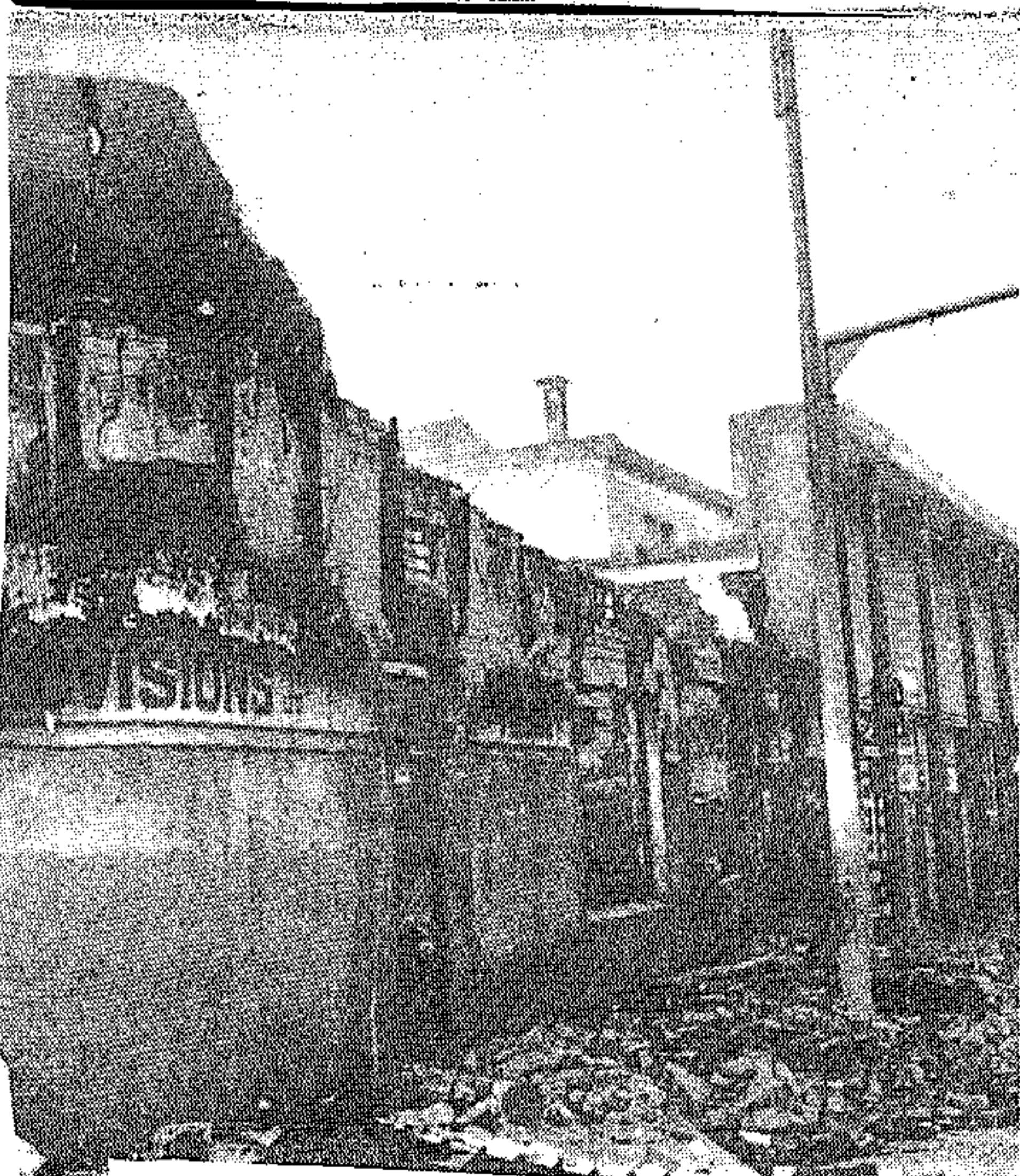
AFTERMATH: A scene of destruction
