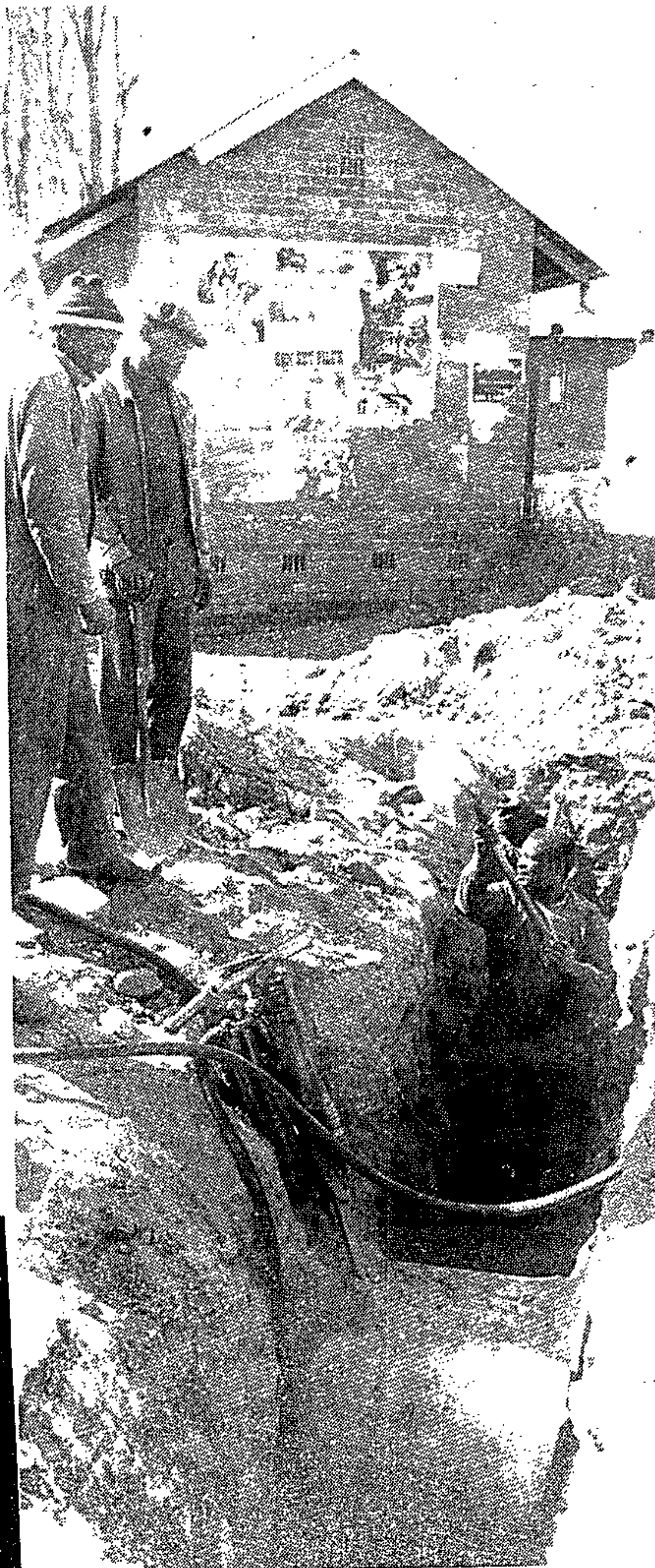
Another trench for electric cables and storm water drain pipes.
