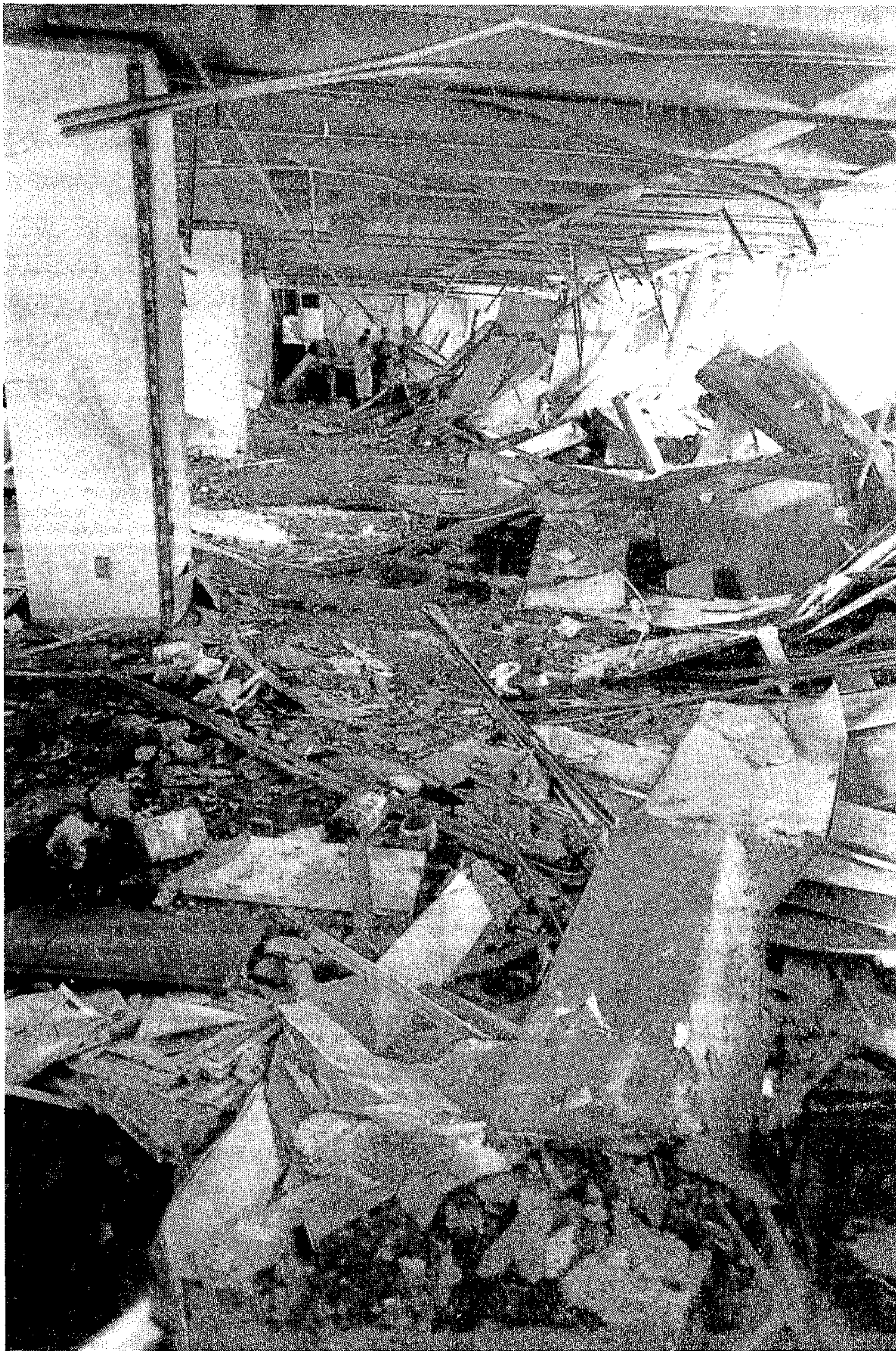
Destruction at 320 West Street during Friday's bomb blast. Virtually everything around the bomb was blown away and pushed up into corners. Even heavy steel safes were whipped aside.
