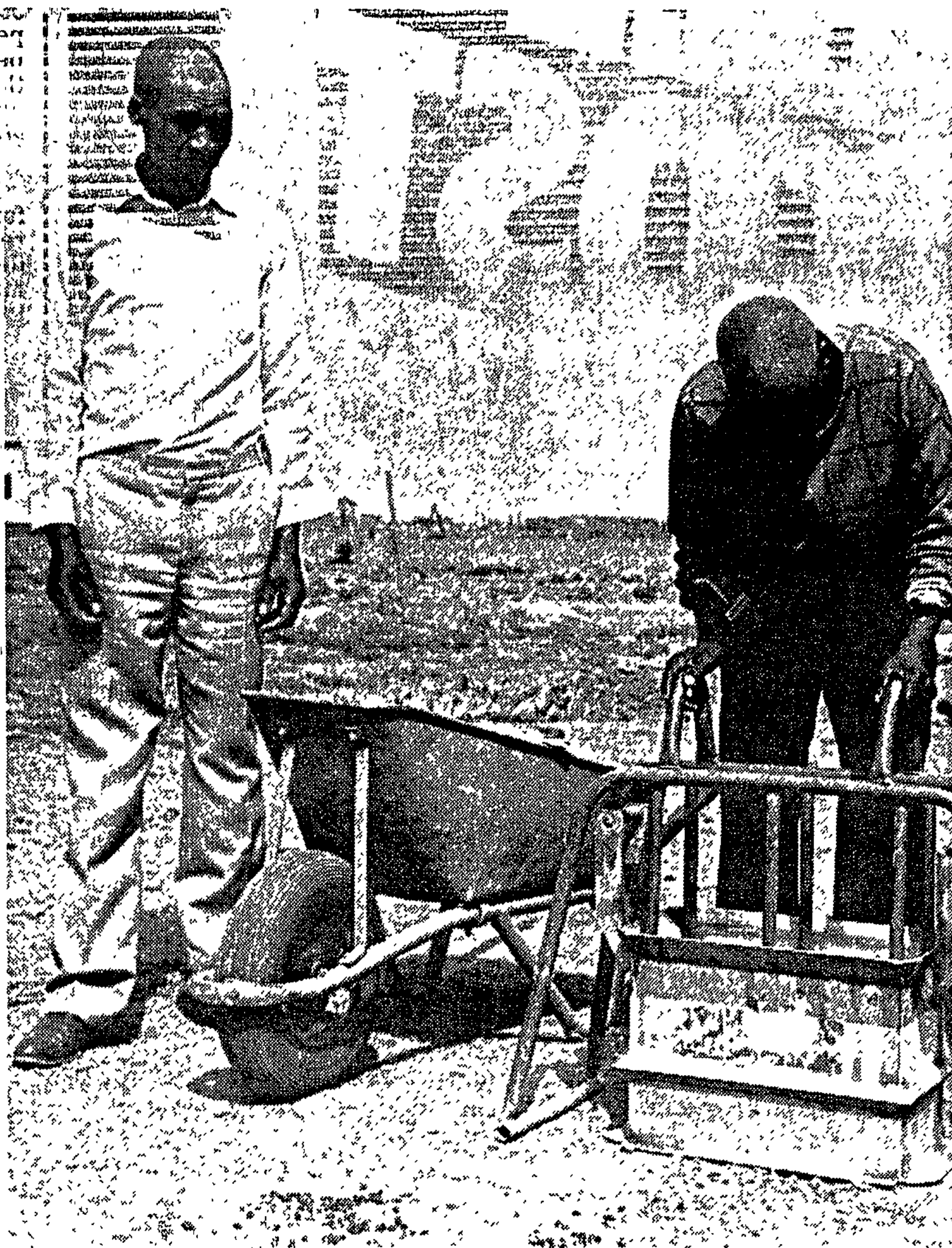
Block-making at Embekweni, a project for improved housing and producing about 80 blocks a day.
