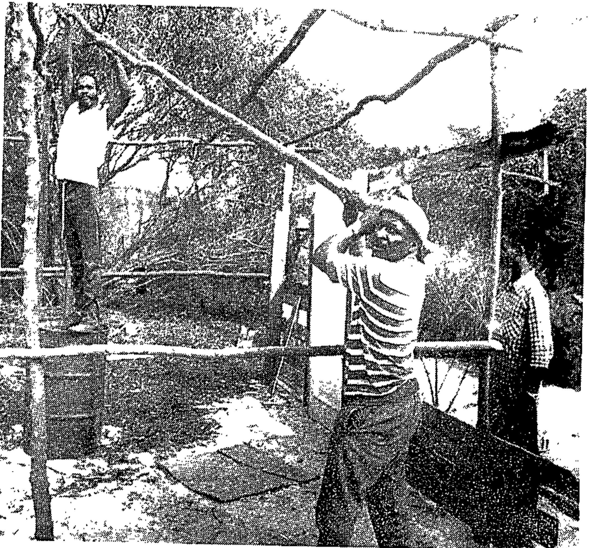
HEAVE-HO . . . Mr Joseph Themba Ntswangela (foreground), helped by Mr Zulungle Vityolo, builds a shack in Noordhoek.
