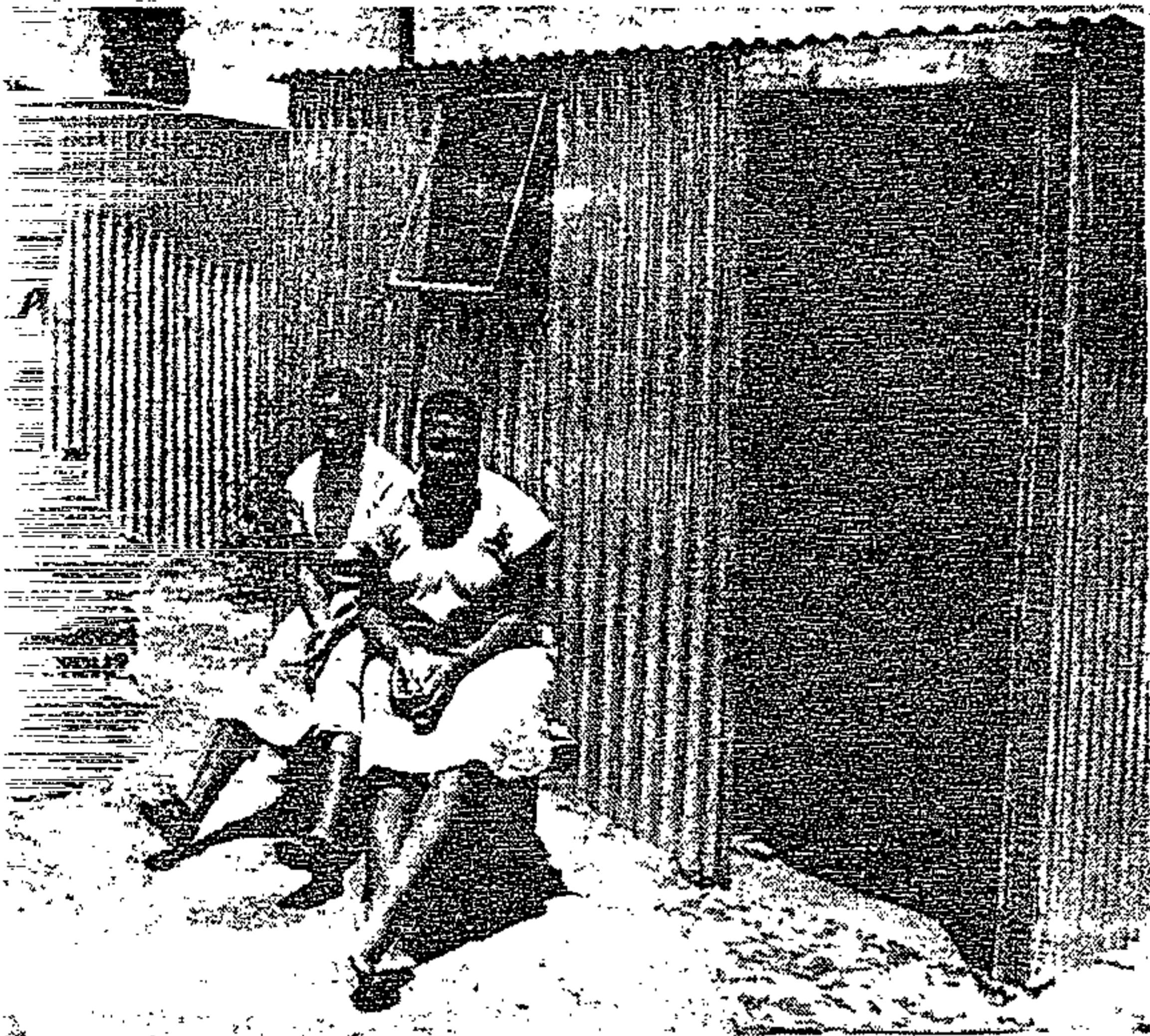
...s have not yet been demolished. Here residents wait for their turn.
