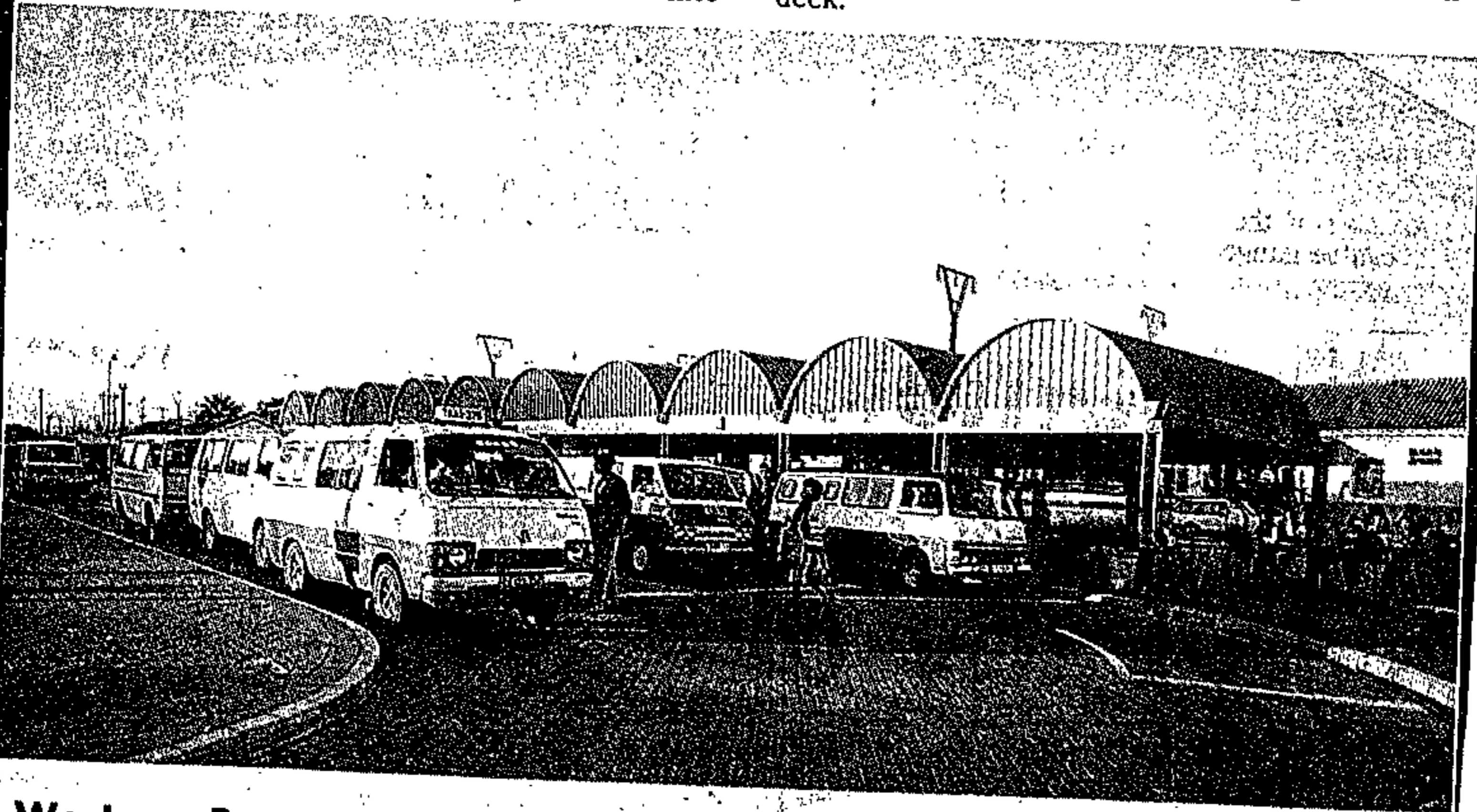
Work on Retreat railway station's rank has made life more comfortable for taxi users, but the shelter covers mainly bus commuters.
